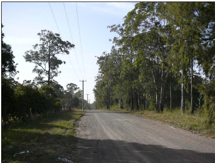
Photo 4 – General view of Boundary Rd east of Medowie Rd.
